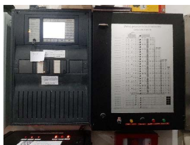
Graphic Annunciator Fire Alarm System
