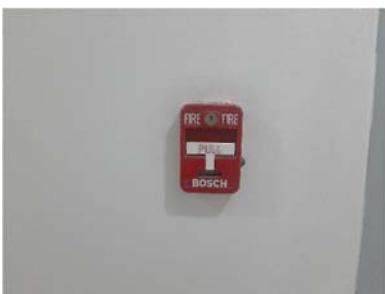
Fire Alarm Manual Station
