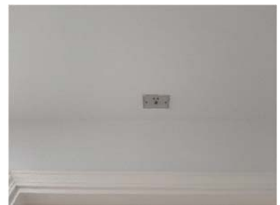
Fire Alarm Indicator Lamp
